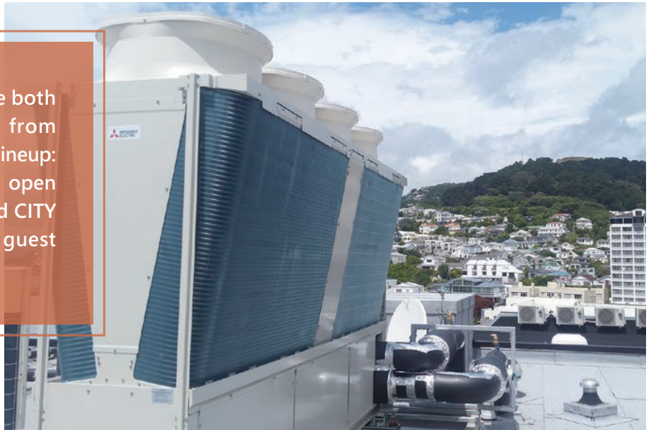
Rooftop installation of the e-series
