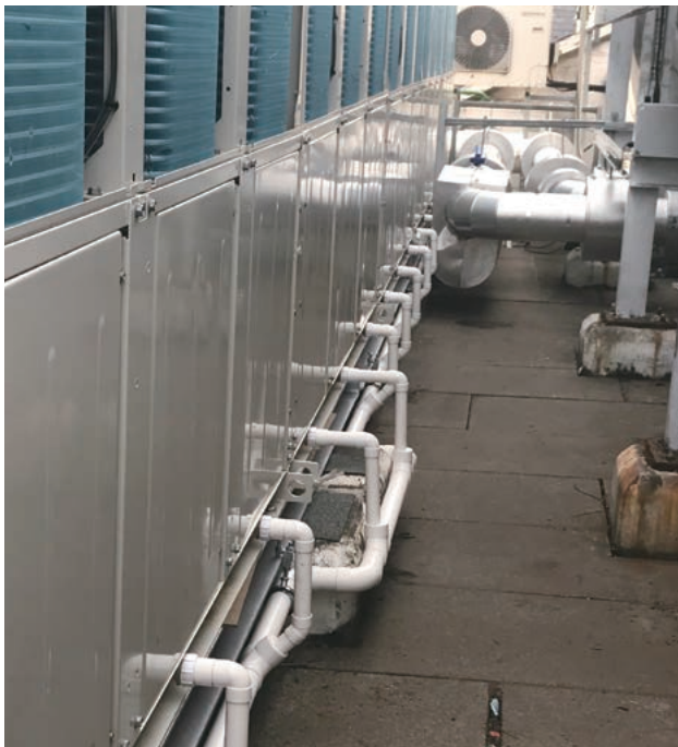
Built-in header piping can reduce space and make water piping work simple.
