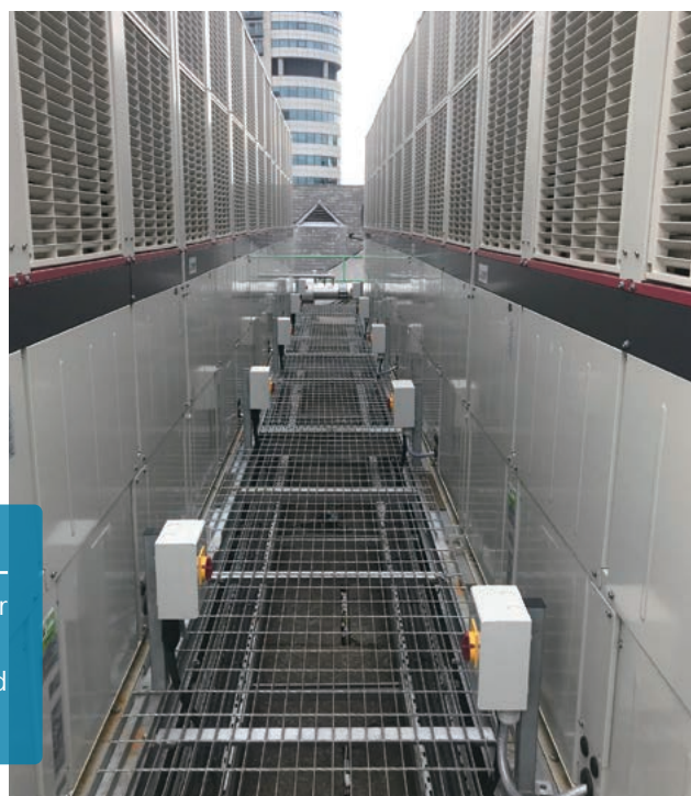
Built-in header piping can reduce space and make water piping work simple.
