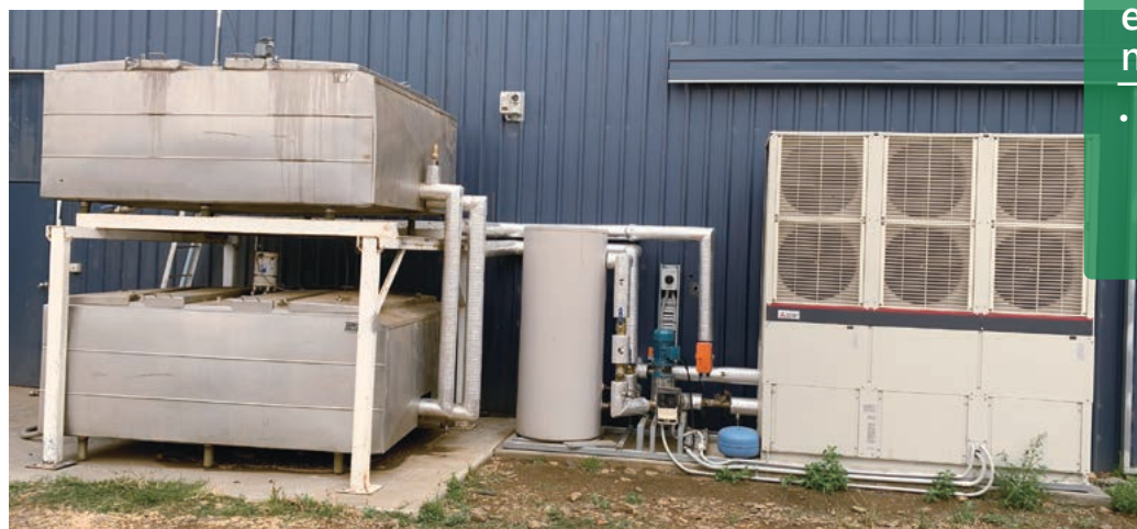
e-series, buffer tank and calf milk vat 1&2 (from right)
