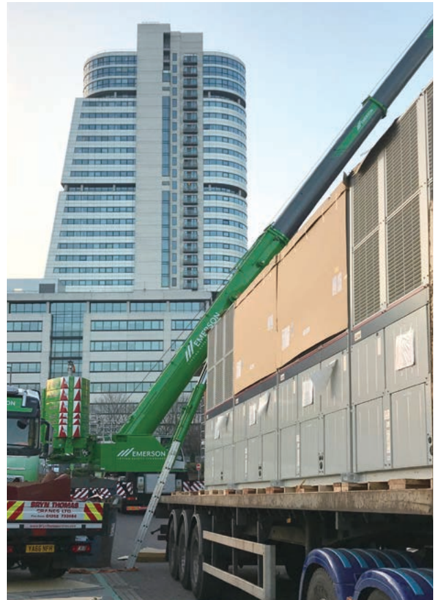
e-series delivered to site, carried to the rooftop with a crane.
